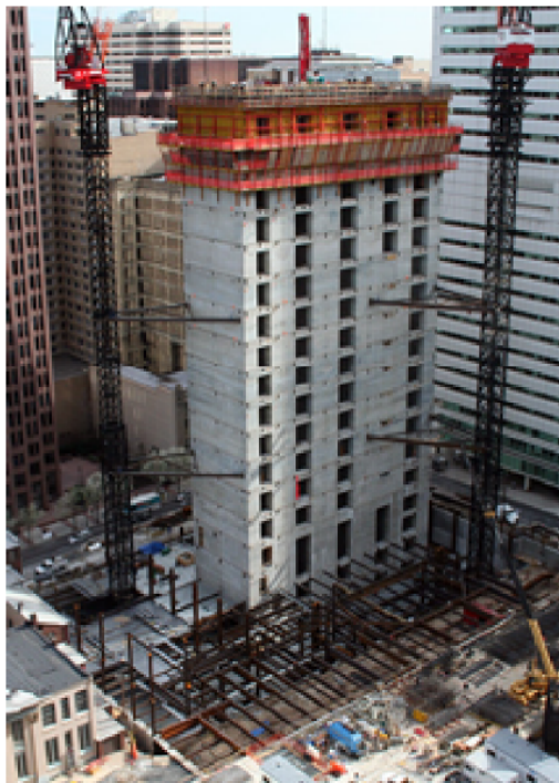
FIGURE B-5: CONCRETE CORE CONSTRUCTED FIRST, STEEL ERECTION FOLLOWS
